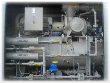
There was an immediate temperature drop averaging 15-20°F (8-11°C) cooler than with the commercial grade product. The lower temperature has stayed consistent since that time. Tom also noticed that the Monolec 1282 flowed better through the drain port than the commercial product that clumped out. The bearing failures have been eliminated since the conversion to Monolec 1282.
